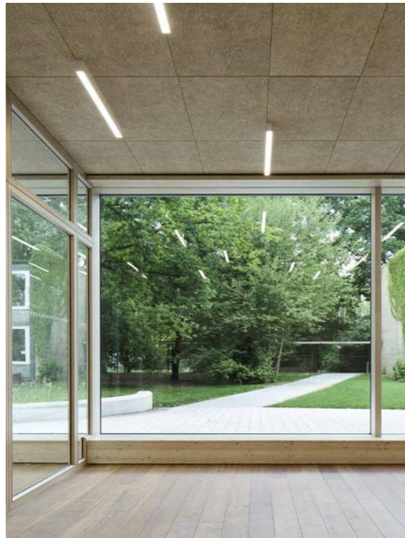
Moabitler Kinderhof (Moabit Children's Court) designed by Kersten Kopp Architekten
