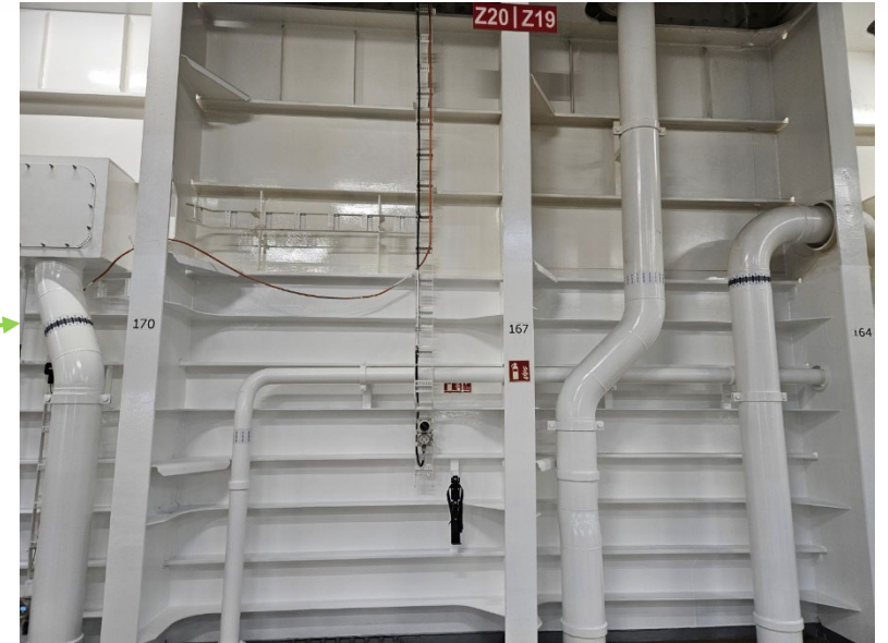
Deck 5 – steel work and painting complete
